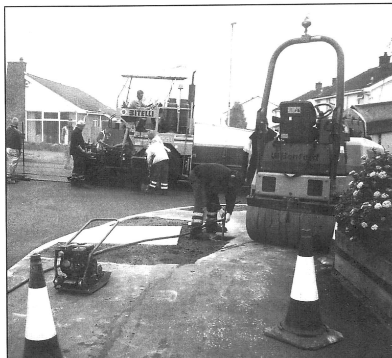
Work underway on Danehill to install one of a series of speed tables, part of the Traffic Calming Scheme.
